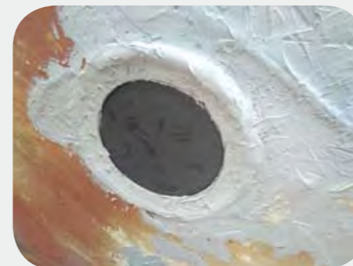
New anode installed
