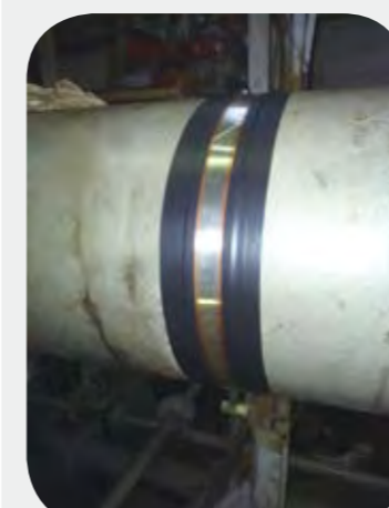
New S.E.D. installed
