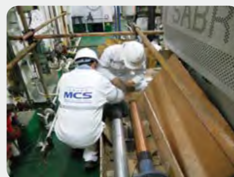
New MGPS electrode assembly
