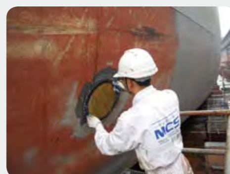
ICCP anode renewal work in Dry-dock
