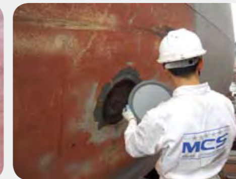
ICCP anode renewal work
