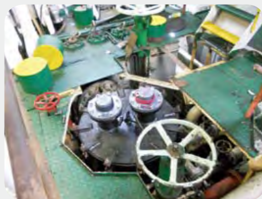
MGPS anodes mounted on strainer's lid
