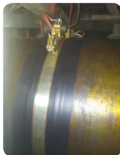
New set S.E.D. installed
