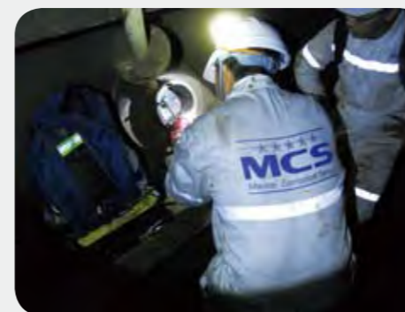
Anode renewal work in the tank
