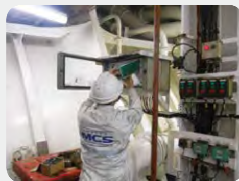
Inspection & repair on MGPS panel
