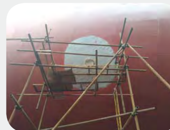
Di-electric shield applied
