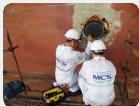
ICCP anode inspection
