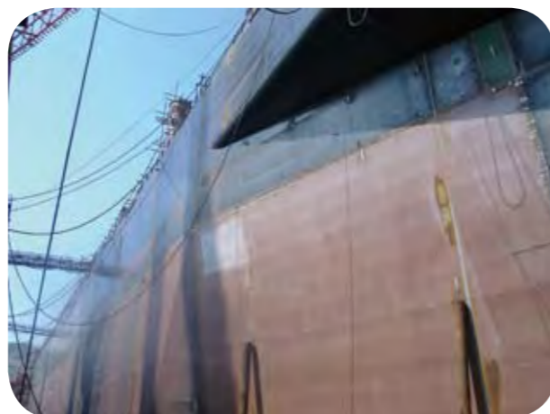
Hull conditions with ICCP system working
