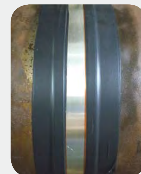
Slip ring installed
