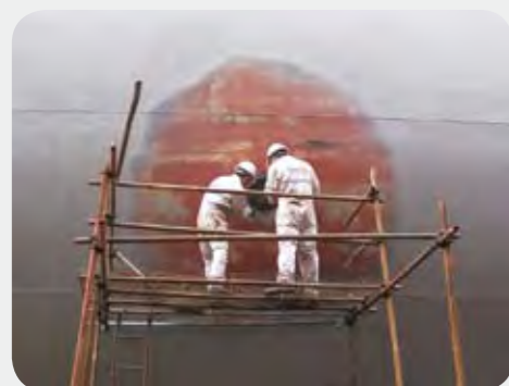
ICCP anode renewal work
