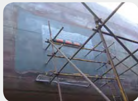
ICCP Linear anode renewal work
