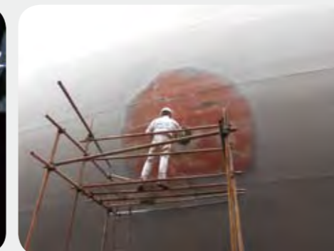
Maintenance and repair work on the Di-electric shield
