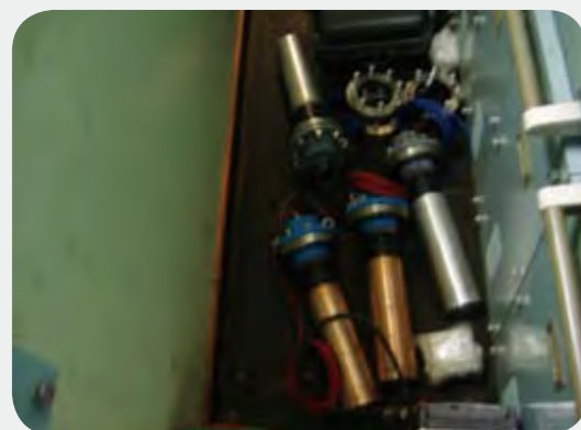
New MGPS anode assembly
